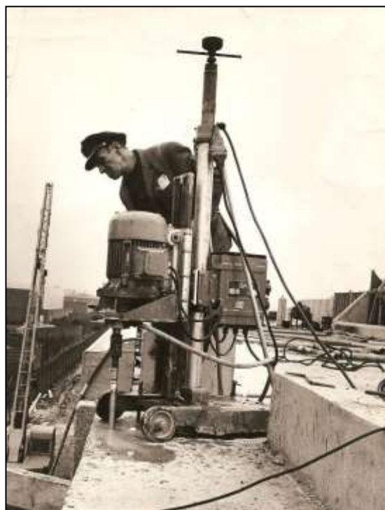
Cor, boren in beton
